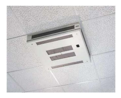
The heater appliance is designed to fit either directly to the ceiling or suspended through a 600mm x 600mm tile surround. The MAXIMUM recommended height from floor to underside of unit must not exceed 3.2 metres. When installing in a suspended ceiling the appliance must be supported by chains or threaded rods. Do not attempt to fix the unit to the ceiling tile frame.
