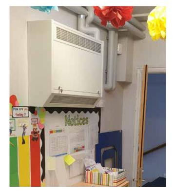
Warm air is discharged at an upward 45° angle to avoid causing discomfort to people sitting adjacent to appliance and with chamfered profile to avoid sharp corners
