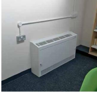
Fan convectors are ideal for schools because they are compatible with all types of wet central heating systems and they function equally efficiently connected to a conventional boiler or to renewable technology, such as biomass boilers or ground or air source heat pumps.
