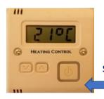
**Step 5:** Press the button to exit pairing and switch OFF
